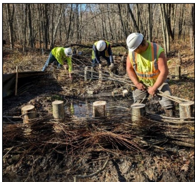
Constructing a mock beaver dam analogue
